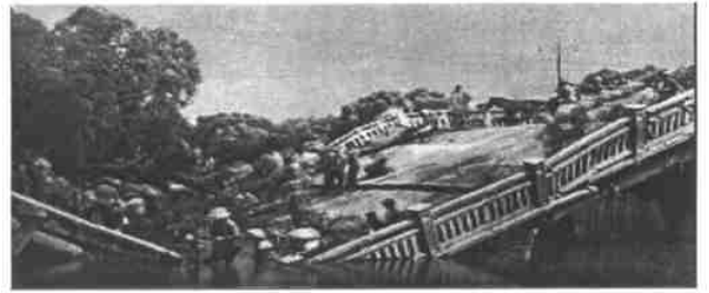
图 1 1976 年唐山地震中胜利桥震害 Fig. 1 Damage of the Victory bridge in the 1976 Tangshan earthquake
