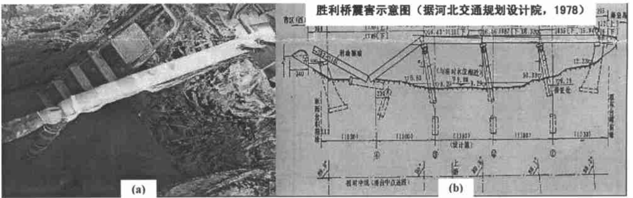
图 7 模型桩与原型桩震害对比 Fig 7 Comparison of seismic damages between model and prototype piles
