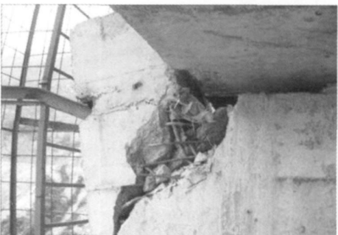
(c) 挡块根部斜向剪切破坏
