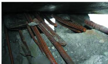
(m) 纵筋节点处绑焊接
